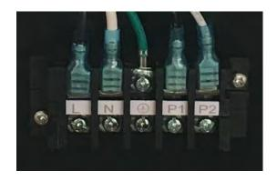
Position L,N and  $\ \ \, \bigoplus$  is for the power connection of our heat pump.
